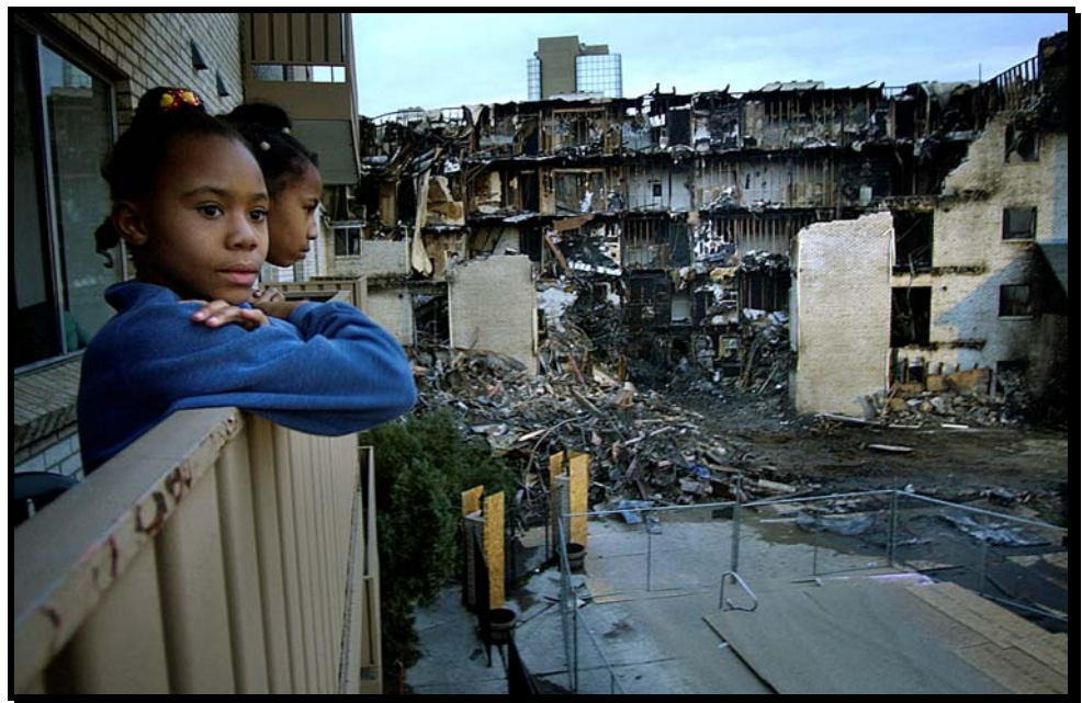
The Spanish Gate fire aftermath, seen from adjacent building. Photo © Evan Semon.
